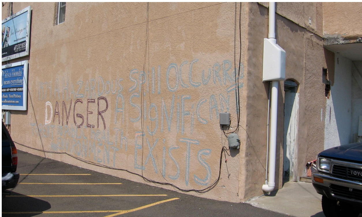
Commercial Building with Vapor Mitigation System
