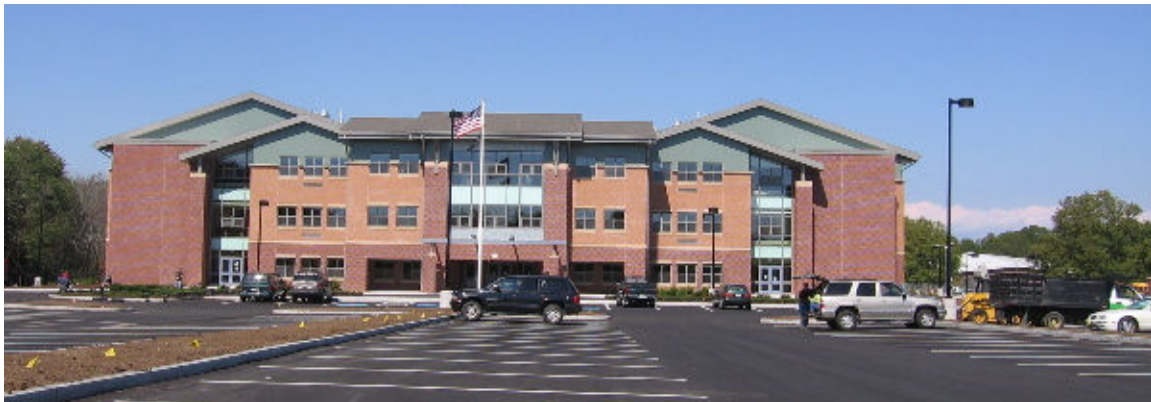
Keith Middle School, built on an old dump in New Bedford, Massachusetts
