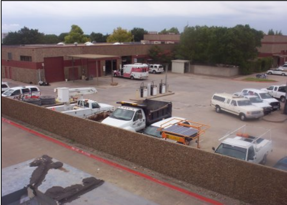
Addison Maintenance Facility to South
