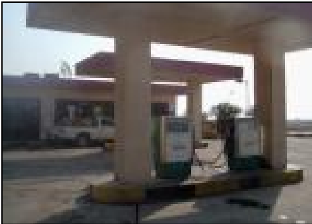
View of dispensers and island.
