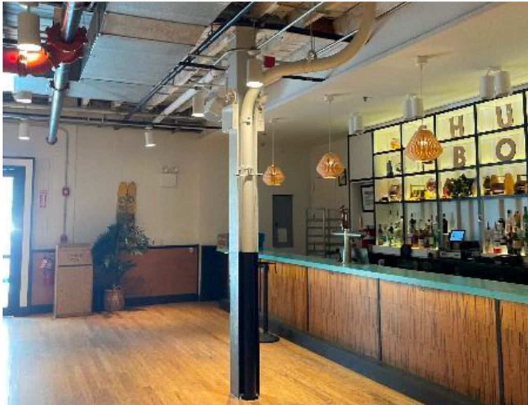
Ventilation Point inside Royal Palms Shuffleboard Club
