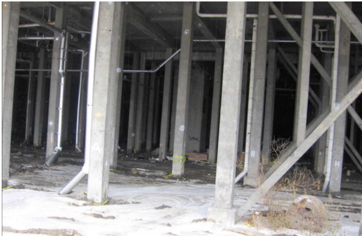
Jet-Grout Waste under P.S. 156
