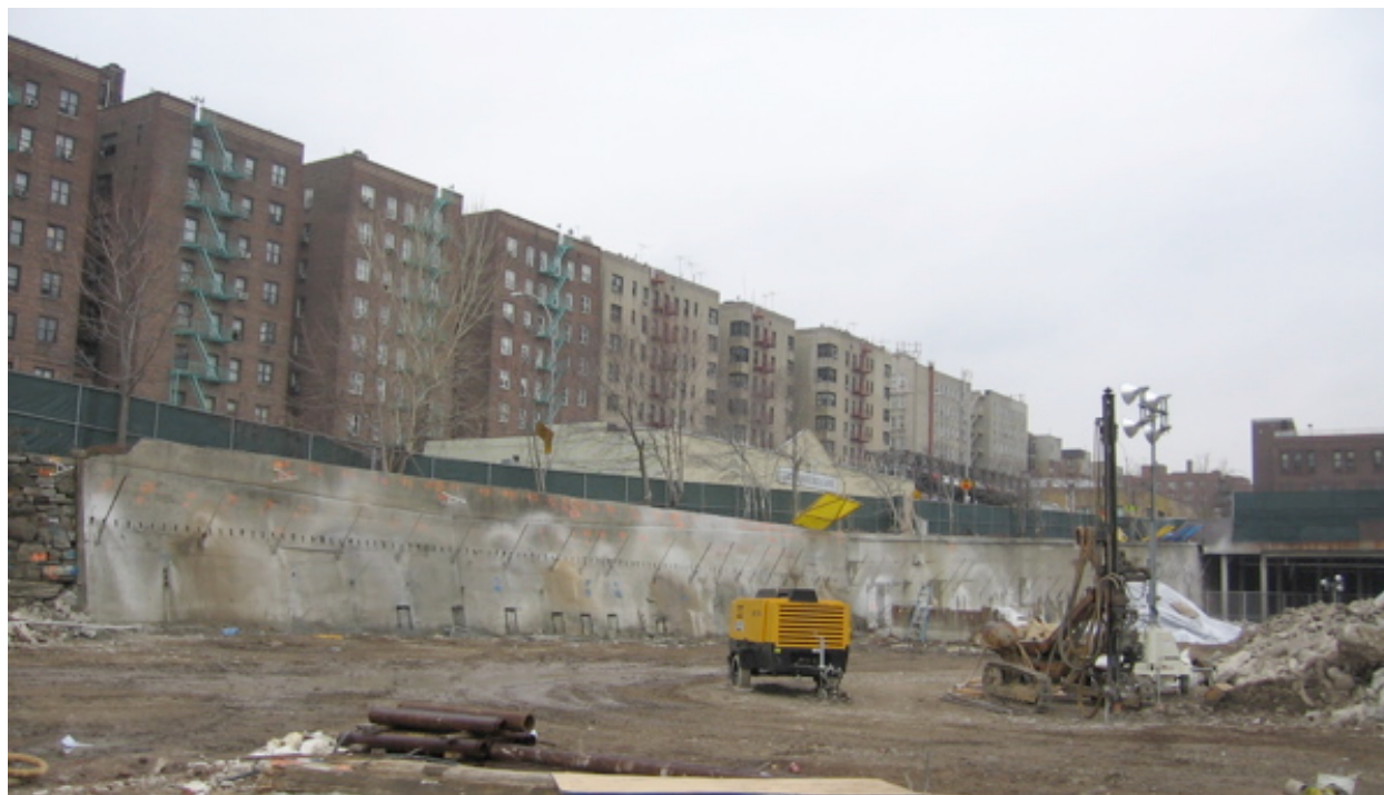
Retaining Wall at Concourse Village West (street)
