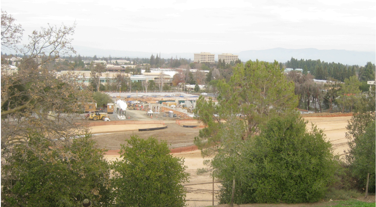
Looking North across 1601 California Avenue
